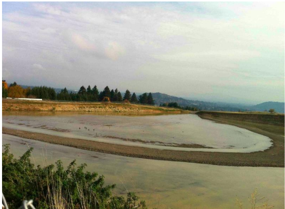
Photo: Excavation site awaits summer construction of the new reservoir.
